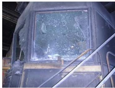
*Figure 1: Pulpit Windows Damaged by Explosion*
