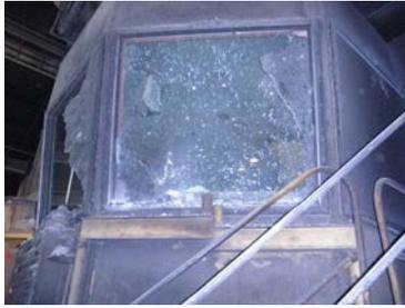
Figure 1: Pulpit Windows Damaged by Explosion
