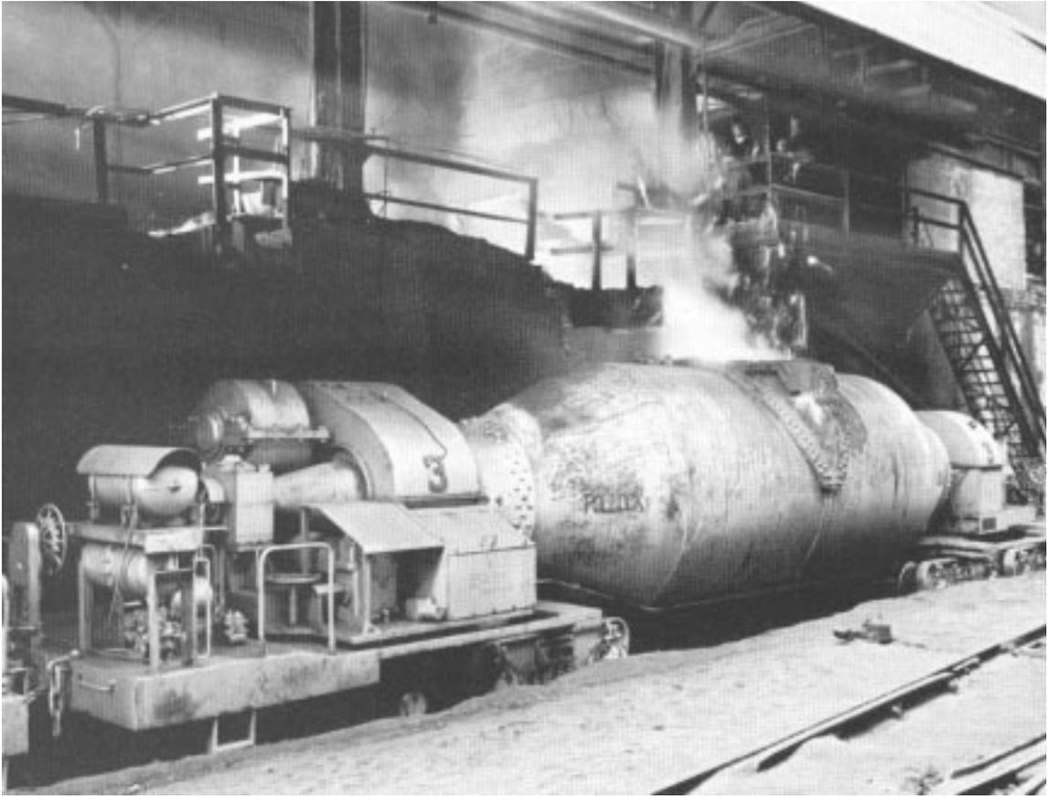
**Fig. 9.55** View of hot metal filling a submarine or torpedo ladle.
