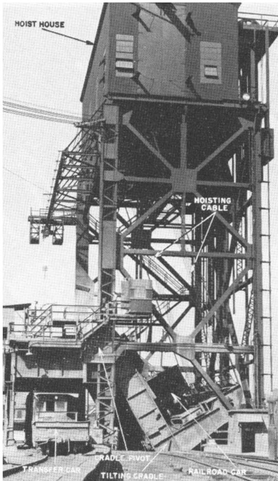
**Fig. 9.42** Car dumper discharging iron ore from a railroad car into a transfer car.
