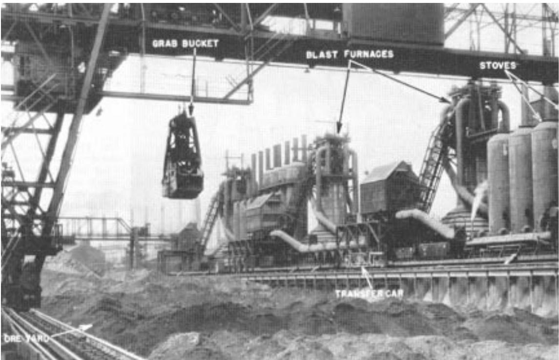
Fig. 9.44 View of an ore yard servicing the blast furnaces in the background.
