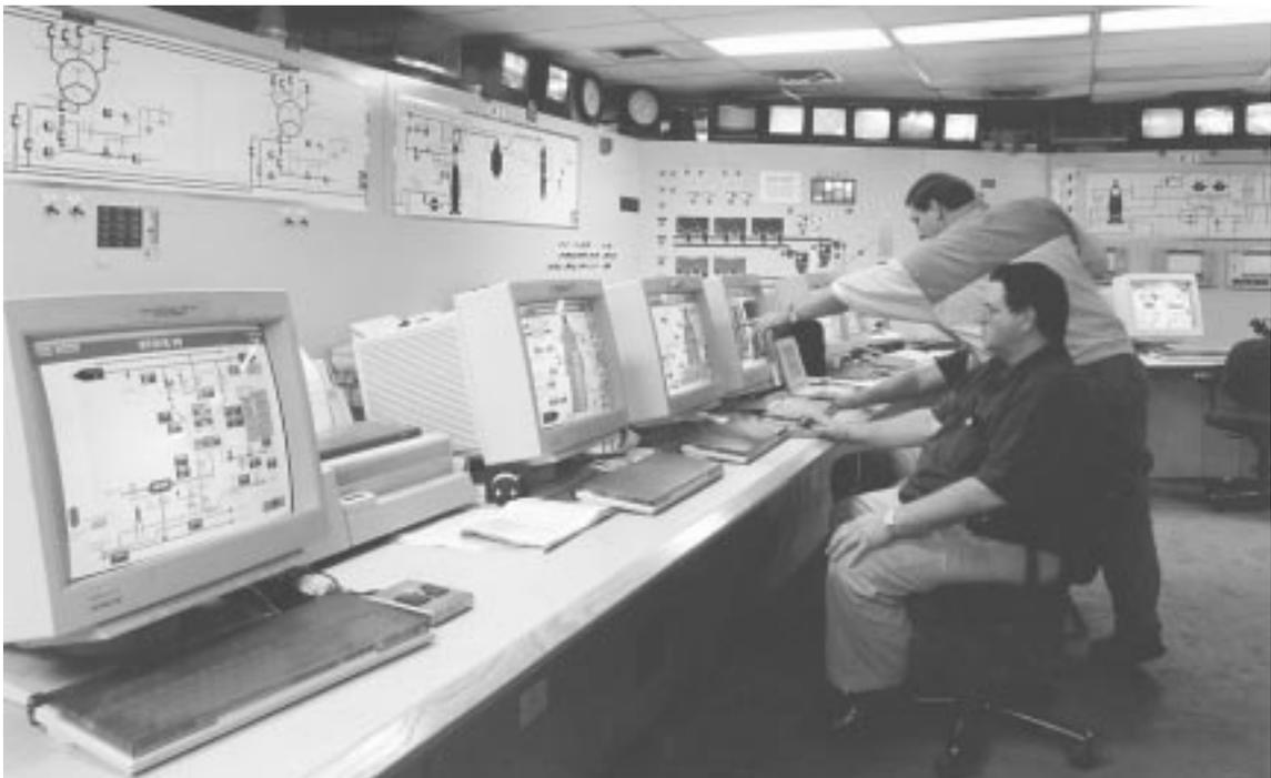
**Fig. 9.58** View of a modern control room with many MMIs for operating the blast furnace. (Courtesy of Kvaerner Metals.)
