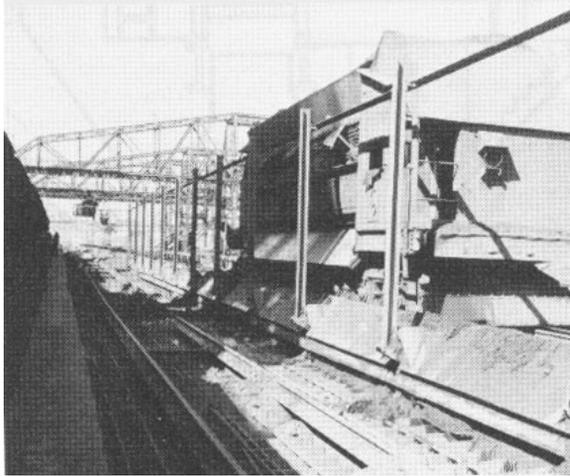
**Fig. 9.45** Transfer or bin car of the side-discharge type shown in position to discharge a load of ore into the stockhouse bins. The ore must pass through the gratings shown, which effectively prevent oversize material from entering the bins.
