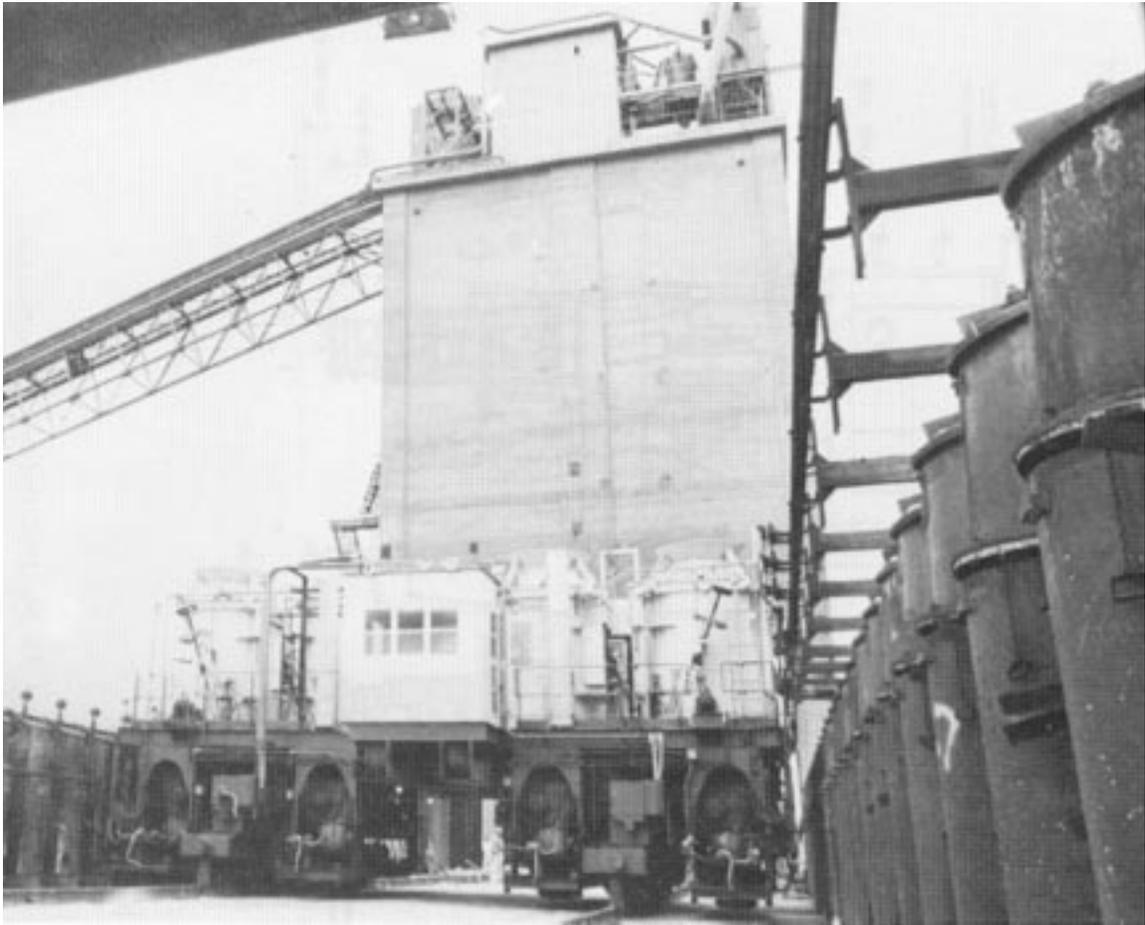
**Fig. 7.37** View of a coal storage bin and larry car on top of a modern coke oven battery equipped with a double collecting main.
