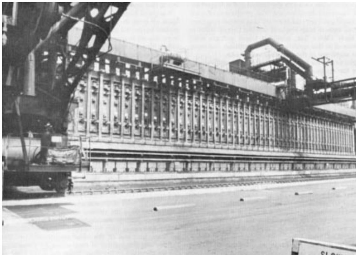
**Fig. 7.22** Overall view of the pusher side of a typical byproduct coke oven battery.
