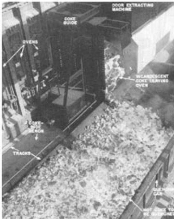
**Fig. 7.43** Coke side of a battery of byproduct coke ovens during the process of pushing the coke out of one of the ovens. The quenching car is self-propelled, and carries the coke to a quenching station where it is sprayed with water before being dumped on the coke wharf.
