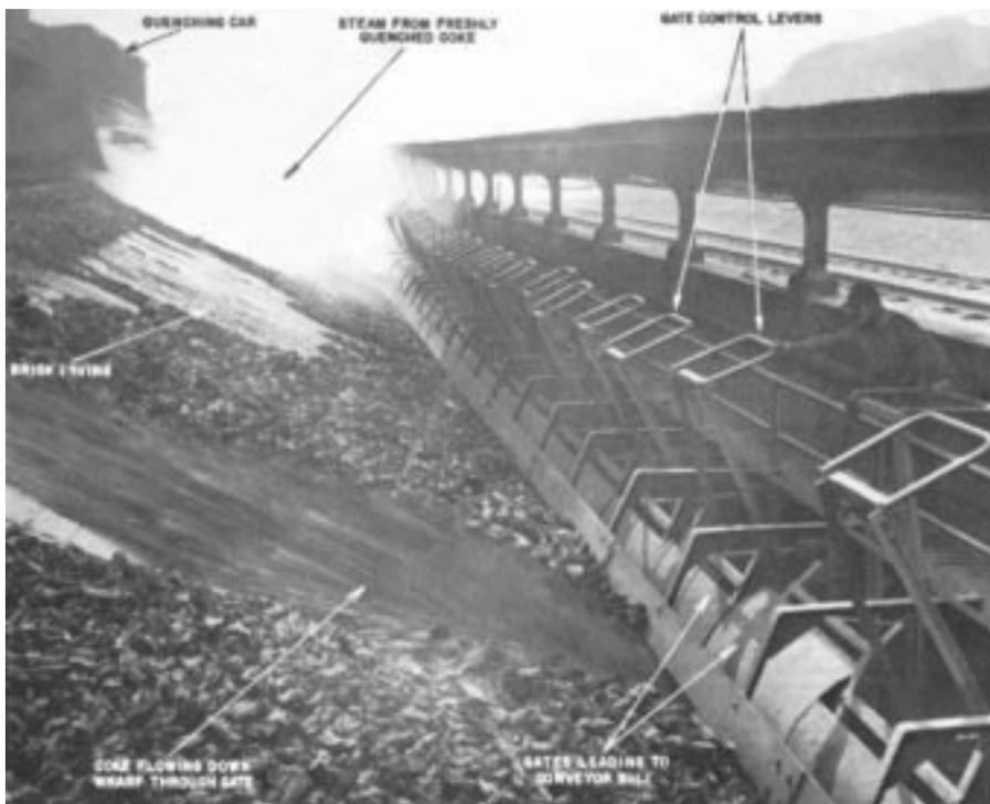
**Fig. 7.49** General view of a manually-operated coke wharf showing freshly quenched coke being discharged from the gates of the quenching car onto the brick paved sloping wharf. When the wharf gates are opened, coke slides down the wharf as at the lower left onto a conveyor belt that carries it to the screening station
