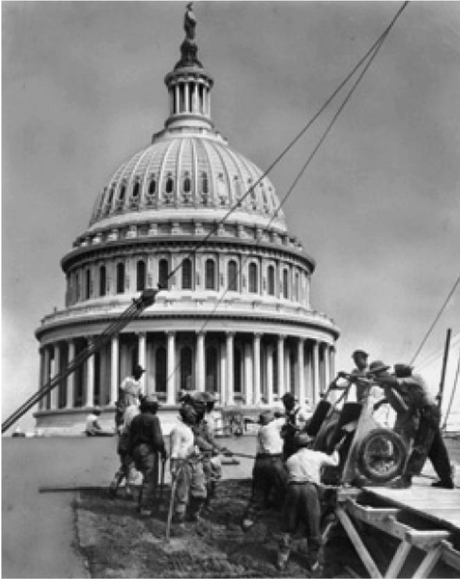
**Figure 10.10** Concrete replacement with LWA structural concrete on the roof of the U.S. Capitol by Southern Lightweight Aggregate Corporation, later Solite Corporation of Richmond, sometime in 1950s. (Courtesy of Northeast Solite Corporation.)
