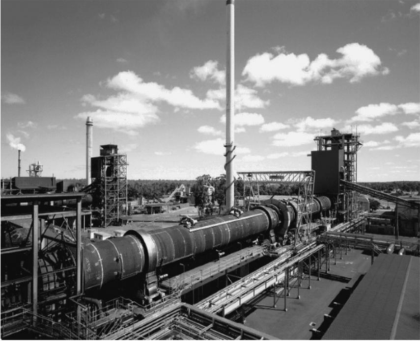
**Figure 10.9** 4.6 by 68 m rotary kiln for direct reduction of ilmenite concentrates with subbituminous coal at Iluka Resources I, Australia built in 1984. Capacity: 900,000 metric tons per year ilmenite feed. (Courtesy of Outotec, Australasia, Pty).
