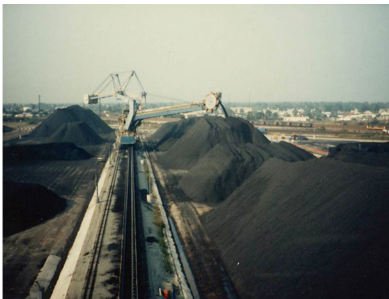
Fig. 1.9 Coke dumping yard
