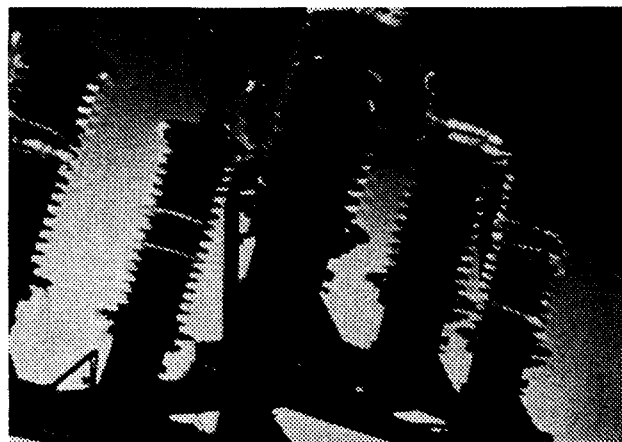
Fig. 8. Similar insulators to Fig. 7 under very severe conditions of arcing in a salt fog with ATH stopping complete breakdown.
