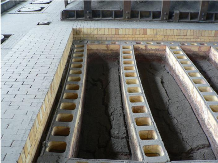
**Fig. 4.2** Deformation of the flue walls
