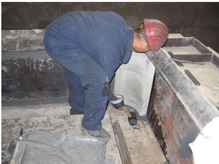
**Fig. 2.76** Installation of the corner SiC block
