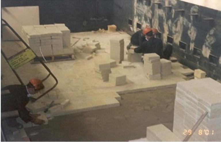
**Fig. 2.84** Lining of the reduction cell: installation of heat insulation vermiculite blocks
