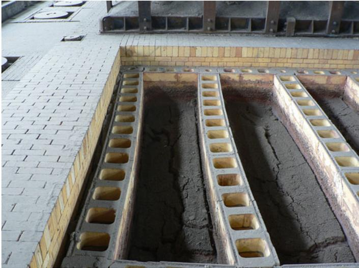
**Fig. 4.2** Deformation of the flue walls
