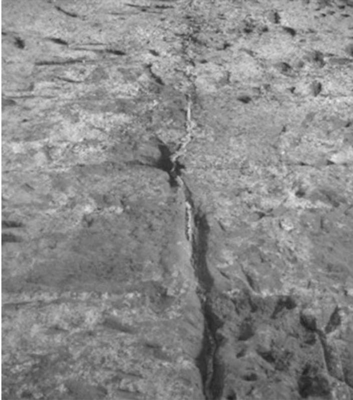
**Fig. 1.11** Crack through the carbon cathode blocks
