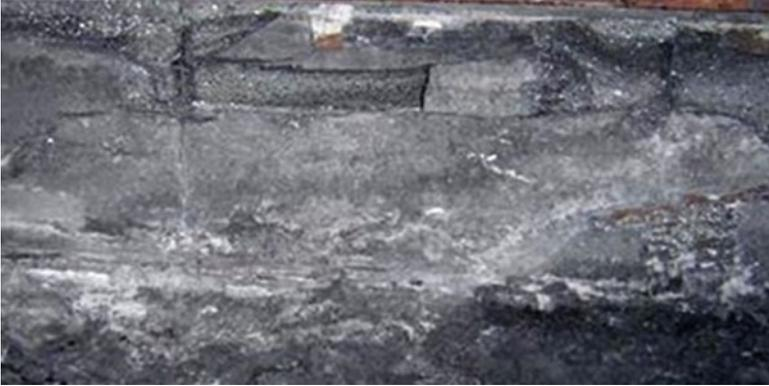
**Fig. 1.26** Cracking in side lining due to strains, caused by oxidation
