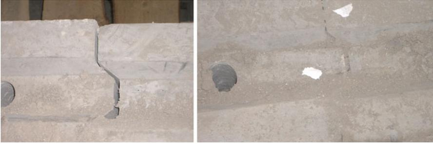
**Fig. 3.14** The temperature gaps between the preshaped concrete blocks
