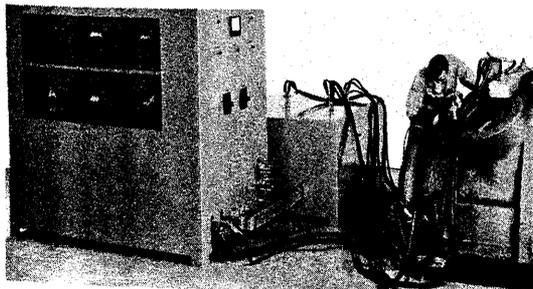
**FIGURE 27. Multidirectional magnetizing of 540 kg (1,200 lb) steel missile forging**
