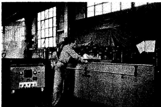
**FIGURE 24. Small wet magnetic particle unit for in-process testing after grinding or heat treating**
