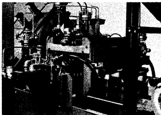
**FIGURE 25. Coupling testing unit using a central conductor for circular magnetization**
