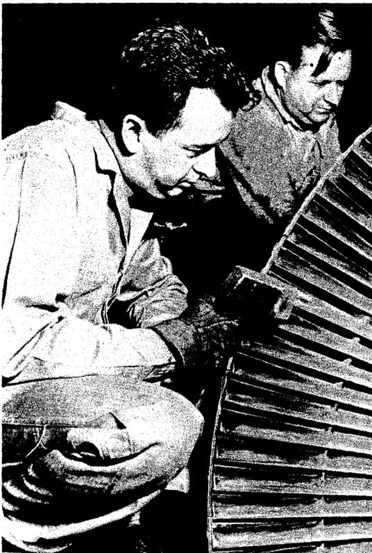
half-wave magnetic particle testing is widely used today for the detection of both surface and near surface discontinuities in welds.
