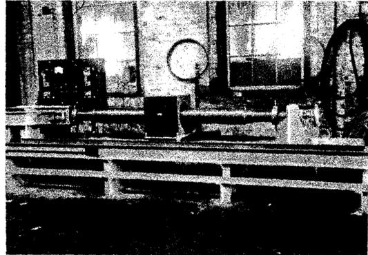
alternating current at diminishing amperages. Larger objects could be demagnetized while still in place on the magnetizing unit.
