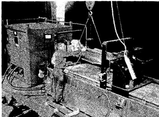
**FIGURE 28. Multidirectional magnetizing system for jet engine blades**
