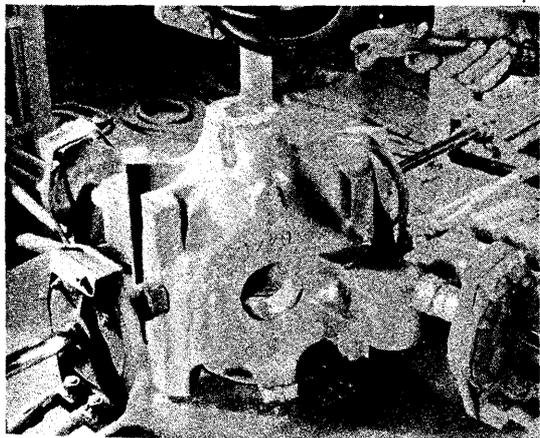
**FIGURE 45. Magnetic particle billet testing using the Ferris wheel**
