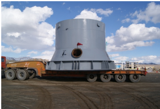
Cooling Gas Scrubber Middle Part
