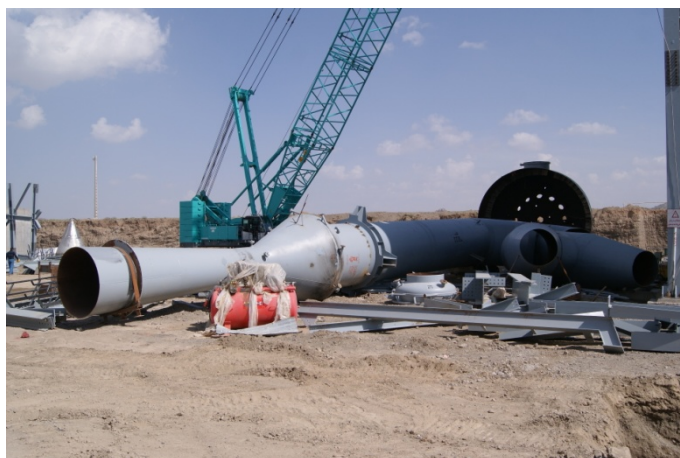
Top Gas Duct
