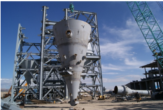
Furnace Lower Parts
