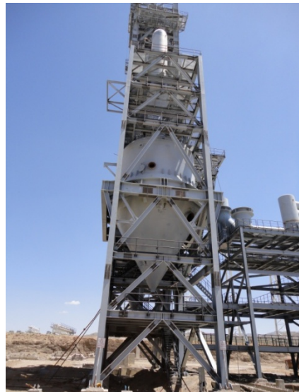
Top Gas Scrubber
