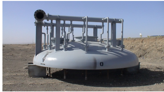
Cooling Gas Scrubber Upper Part
