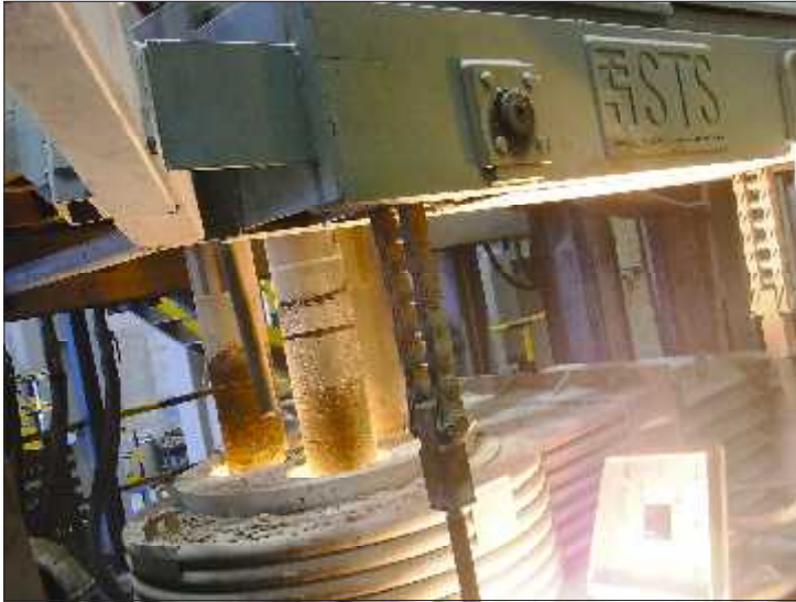
Fig 4 35t ladle furnace
